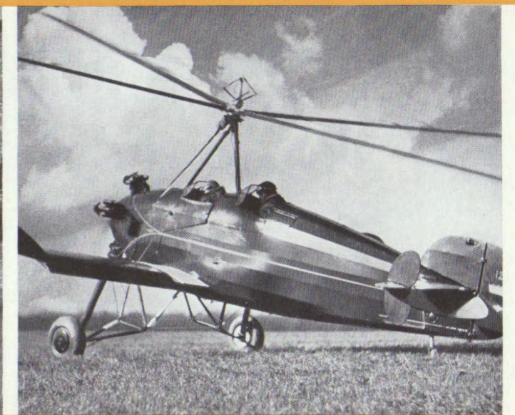
The Pitcairn Tandem, ready to leave the lawn of a country home, with engine and rotor blades started in motion. (Right) Blades have reached take-off speed as shown by the characteristic upward coning position.
